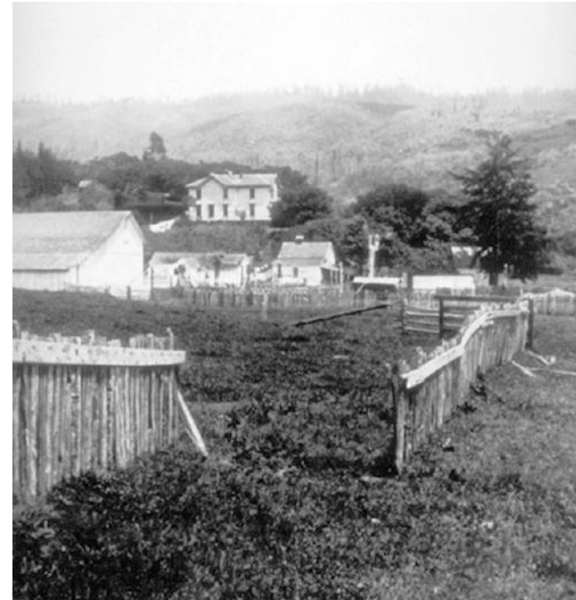
Near Bolinas in Marin County. Picture by G.K. Gilbert showing a fence that was offset about 8.5 feet along the trace of the fault (from Steinbrugge Collection of the UC Berkeley Earthquake Engineering Research Center)
