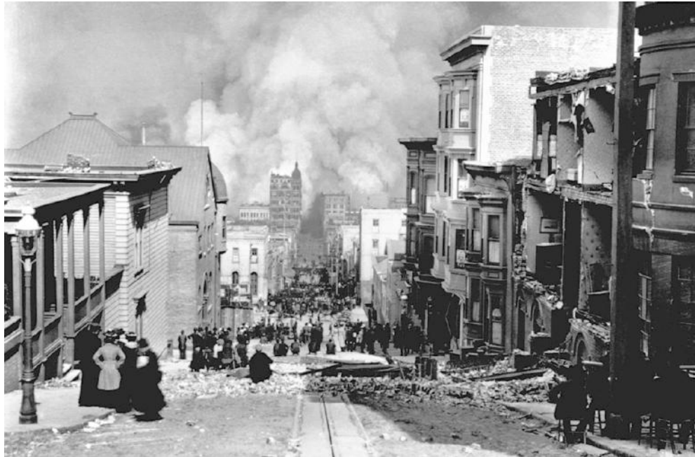
Photograph by Arnold Genthe: Sacramento Street and approaching fire. (Steinbrugge Collection of the UC Berkeley Earthquake Engineering Research Center)
