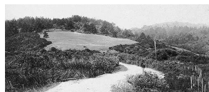
Road to Inverness, California, which had been straight before the earthquake of April 18, 1906, offset twenty-one feet where it was crossed by the earthquake fault. - H.O.W., California Earthquake Investigation Commission. (J. B. Macelwane Archives, Saint Louis University)
