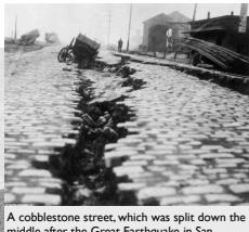
A cobblestone street, which was split down the middle after the Great Earthquake in San Francisco, California, in 1906
