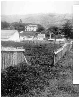
Near Bolinas in Marin County. Picture by G.K. Gilbert showing a fence that was offset about 8.5 feet along the trace of the fault. (from Steinbrugge Collection of the UC Berkeley Earthquake Engineering Research Center)
